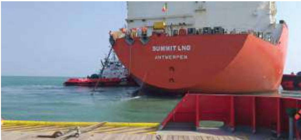
Liquefied Natural Gas (LNG) terminals at Moheshkhali
