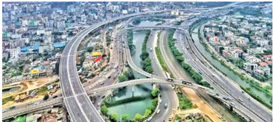
Dhaka Elevated Expressway
